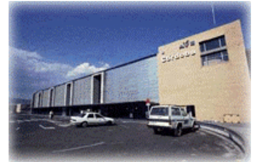
Cordoba railway station
