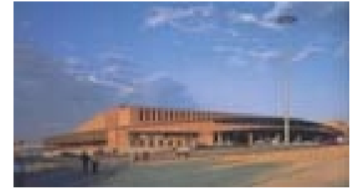
Outside of Sevilla railway station
